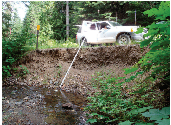
Road survey along Potosi Gulch shows potential for mass failure and sediment contribution to the stream (photo courtesy of USFS).
