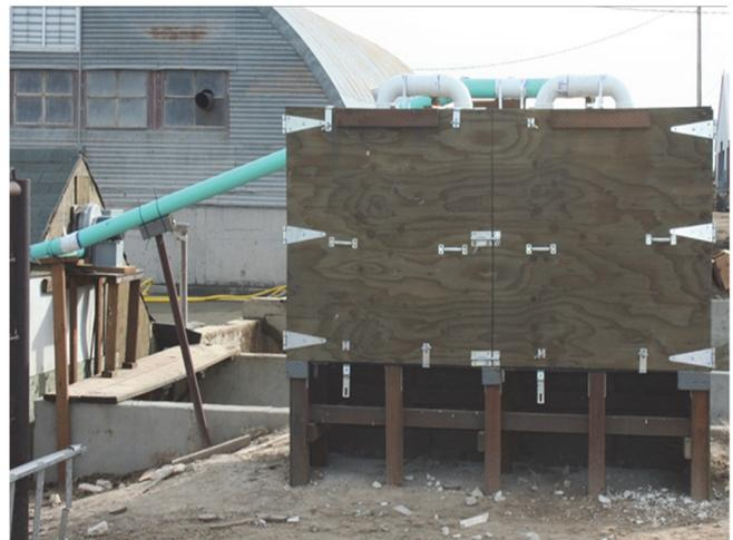
Filter front view, connecting pipe and plenum. Front doors facilitate access, exhaust (bottom); capturing structure (left).
